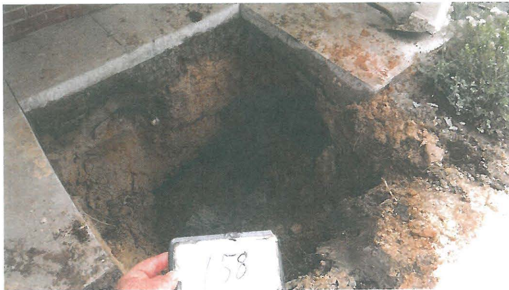
Picture 3: Tank pit.
